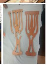
removed the old broken panel, the panel was used as a template to trace onto the new panel.
