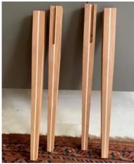
A mortice was cut into the top of each leg to accept the stiffeners. The mortice was cut so that the stiffeners were just 7mm inside the outside of the legs, (That is not in the centre of the legs.)
